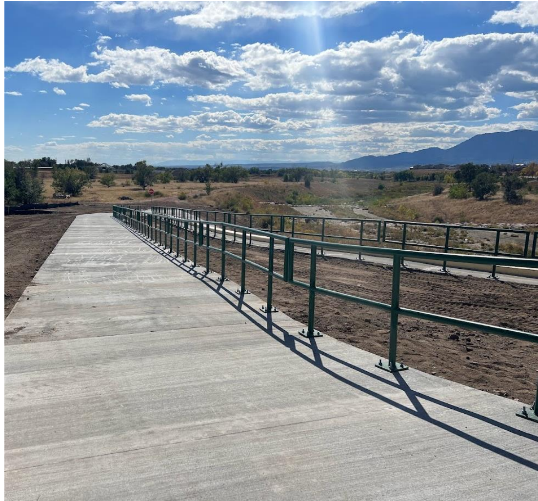
Sand Creek looking south from Platte Avenue: Future Construction
